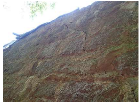
Figure 135 : fissures biaises
